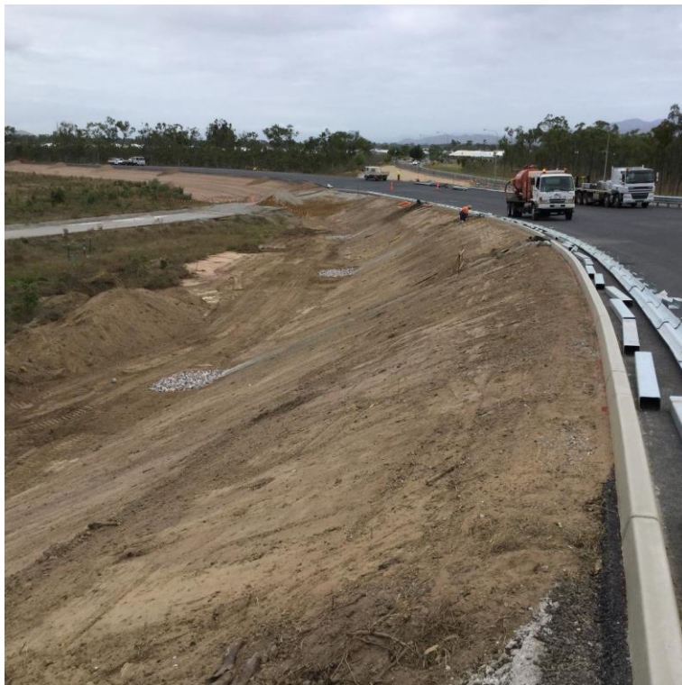
Shaw Rd Overpass batter preparation.
