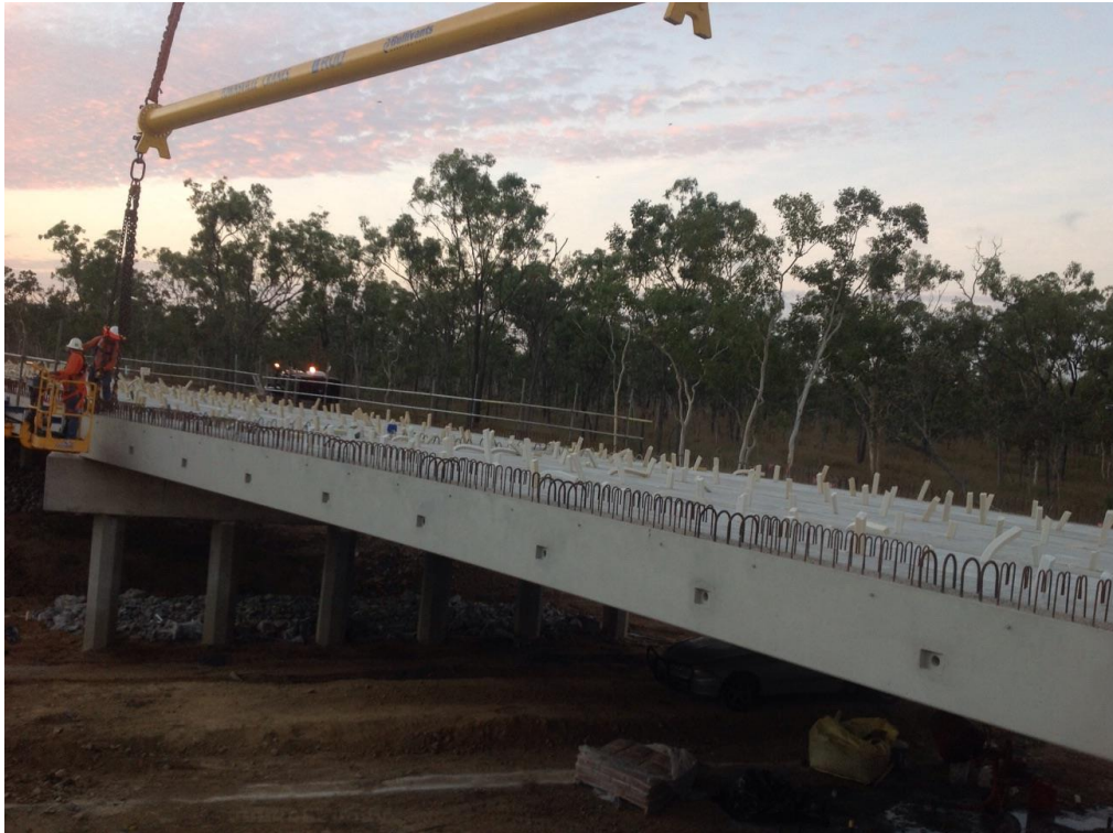
Saunders Ck Bridge.
