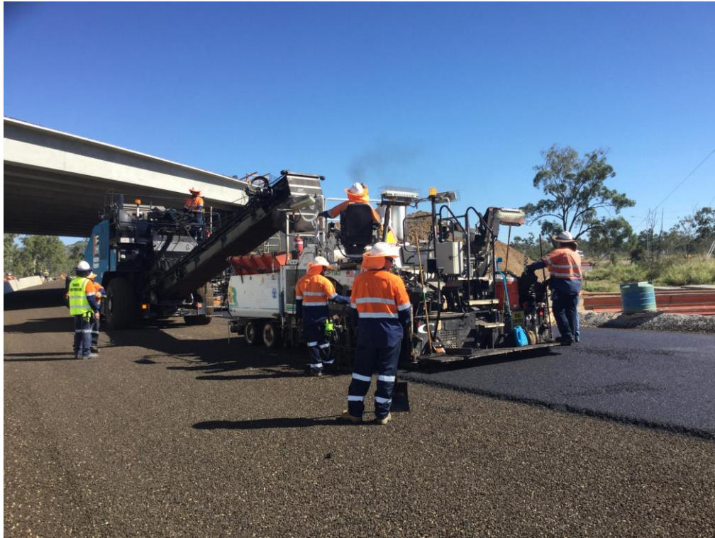
Asphalt Woolcock St
