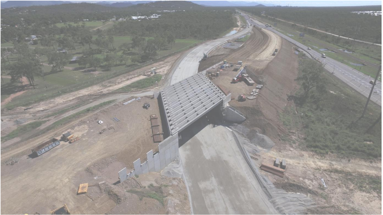
Woolcock St Overpass
