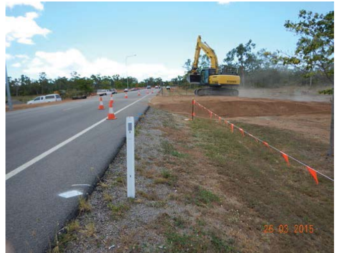
Works on Shaw Road
