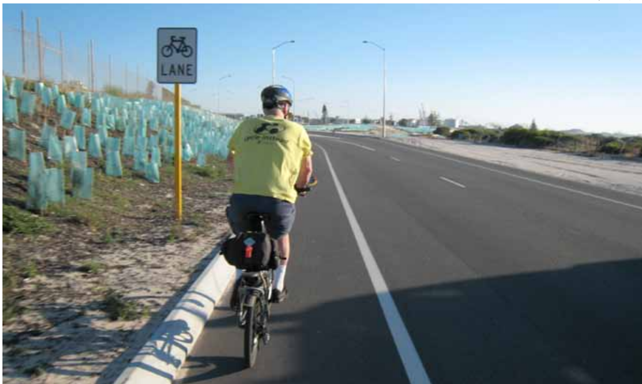
Photo 6: Regulatory sign denoting a bicycle lane near Freemantle, WA. This lane is located beside the kerb on a road without parking.
