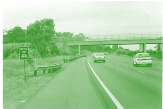
Figure 4 Bike lane/sealed shoulder on multi-lane road
