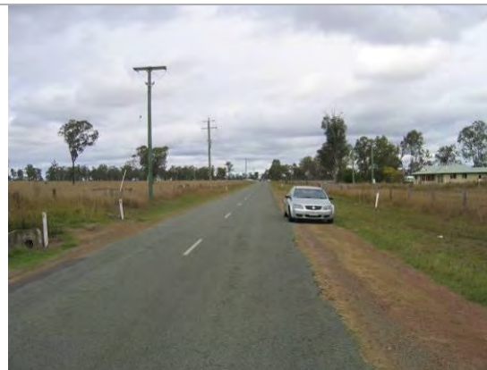
Figure 22 Photo taken in the vicinity of proposed crossing of Middle Road - Road over Rail (Ch 19165)
