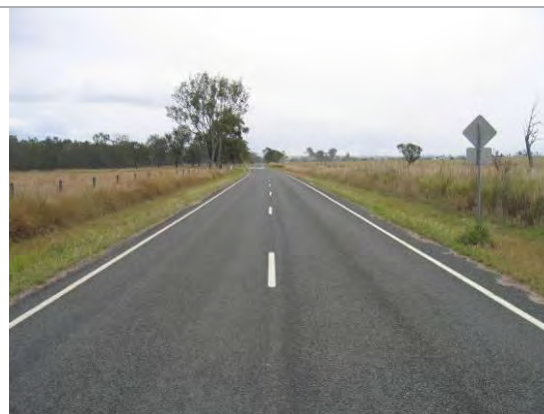
Figure 26 Proposed crossing of Mt Flinders Road - looking west (Ch 25155)
