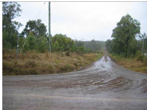
Figure 20 Photo taken from Paynes Road looking south down M. Hines Road (Ch9420)
