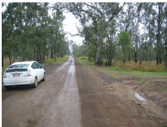
Figure 19 Photo taken looking east along Paynes Road (Ch8450)
