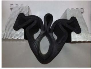
*D* seal glands are not as bulky as *F* seal glands, and can therefore close to zero gap. Refer Figure 18.3-2 *Draped (D) Seal Minimum Closed Gap*.
