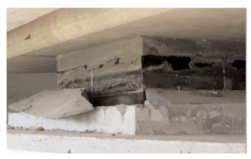
Photo 7: Inadequate fixity around elastomeric bearing
