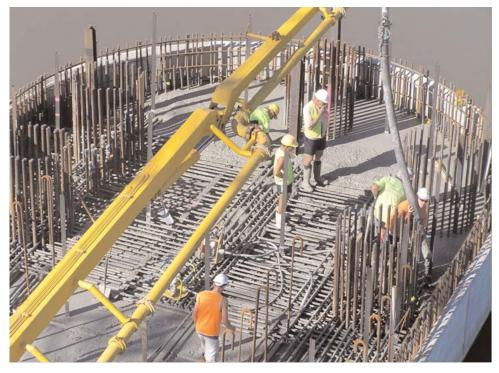
Photo 8: Concrete placement in a pier
