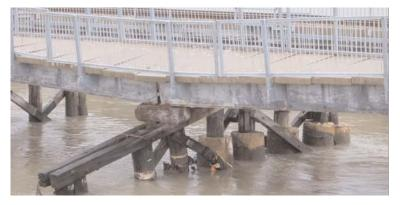
Photo 1: Structural Failure due to degradation of timber piers
