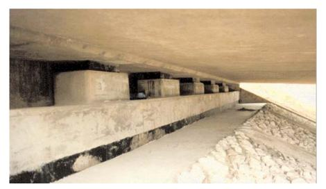
Photo 9: Detailing of bearing shelf, showing bearing plinths and inspection platform
