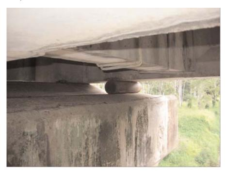
Photo 3: Steel Roller bearings and poor drainage provision on headstock
