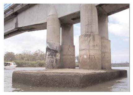
Photo 4: Chloride induced reinforcement corrosion of columns
