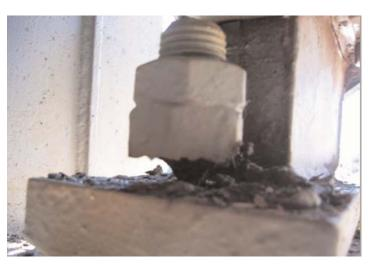
Photo 5: Corrosion resulting in necking of holding down bolt
