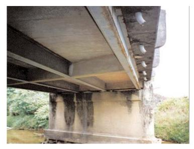
Photo 6: Poor drainage detailing leading to corrosion of outer girder and staining on pier.
