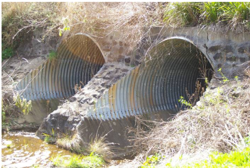
Figure 3.1.1.1 – Multi-plate culvert
