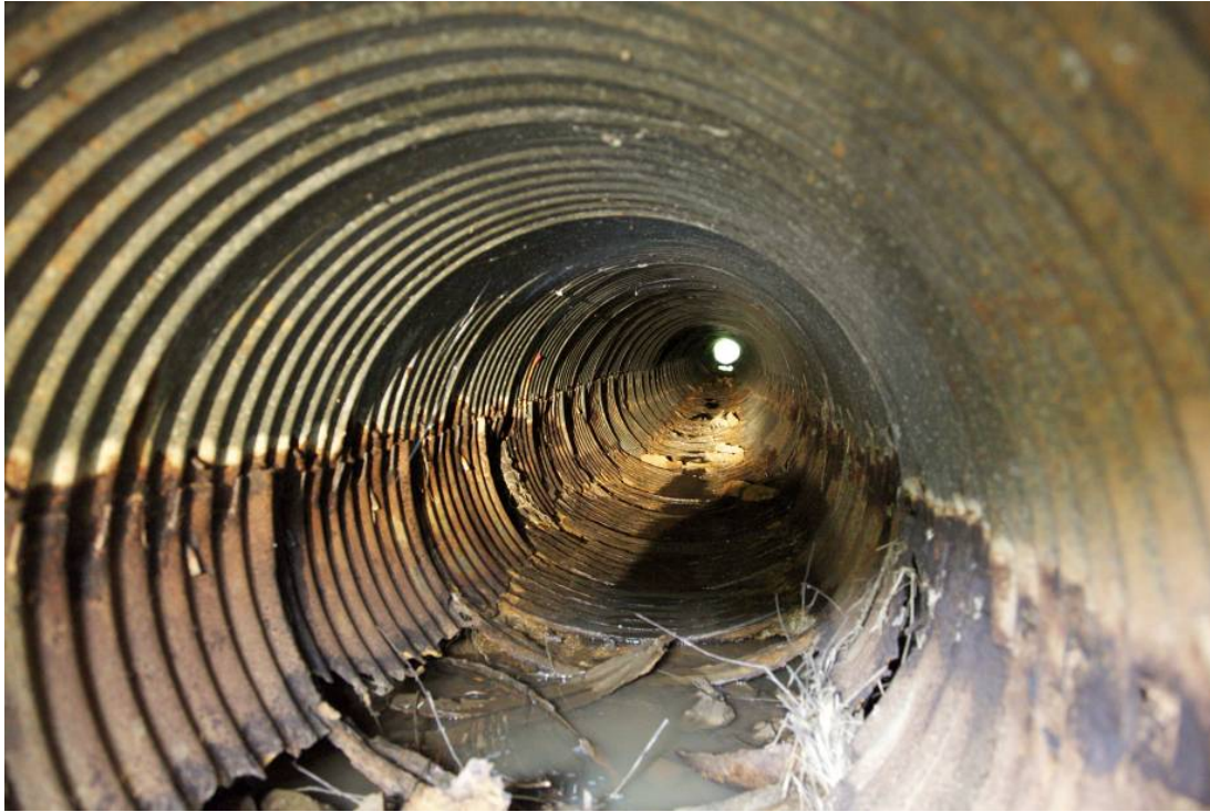
Figure A3 – A culvert exhibiting perforations due to corrosion to the upper portion of the culvert
