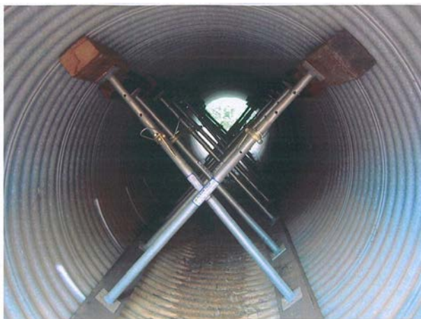
Figure 4.2 – Example of emergency propping
