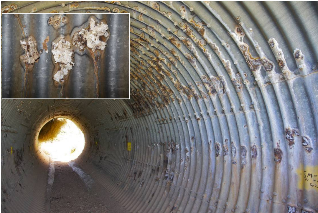
Figure A3 – A culvert exhibiting perforations due to corrosion to the upper portion of the culvert
