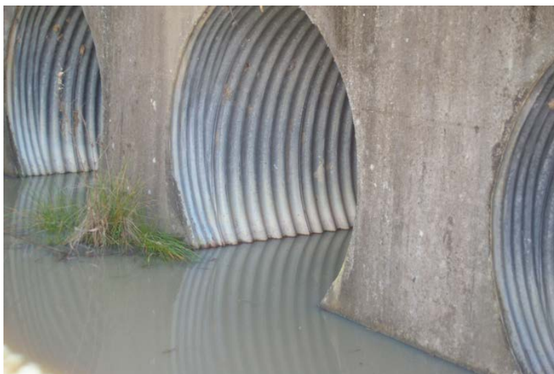
Figure 3.1.1.2 – Helically wound culvert
