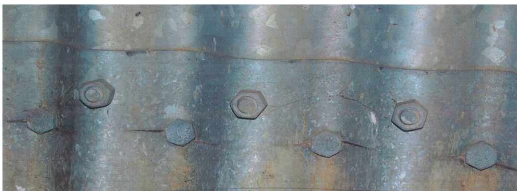
Figure 3.1.8.2 – Cracks in metal plate (Source: ConnDOT, 2000)
