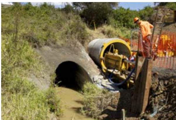
(a) thrust block and hydraulic rams
