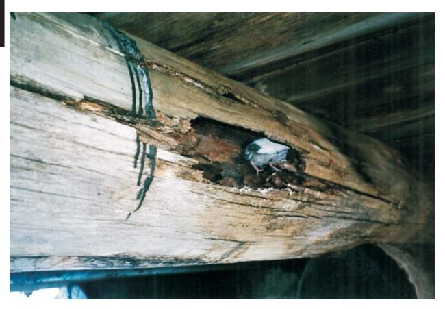
Severe rot hole in girder side
