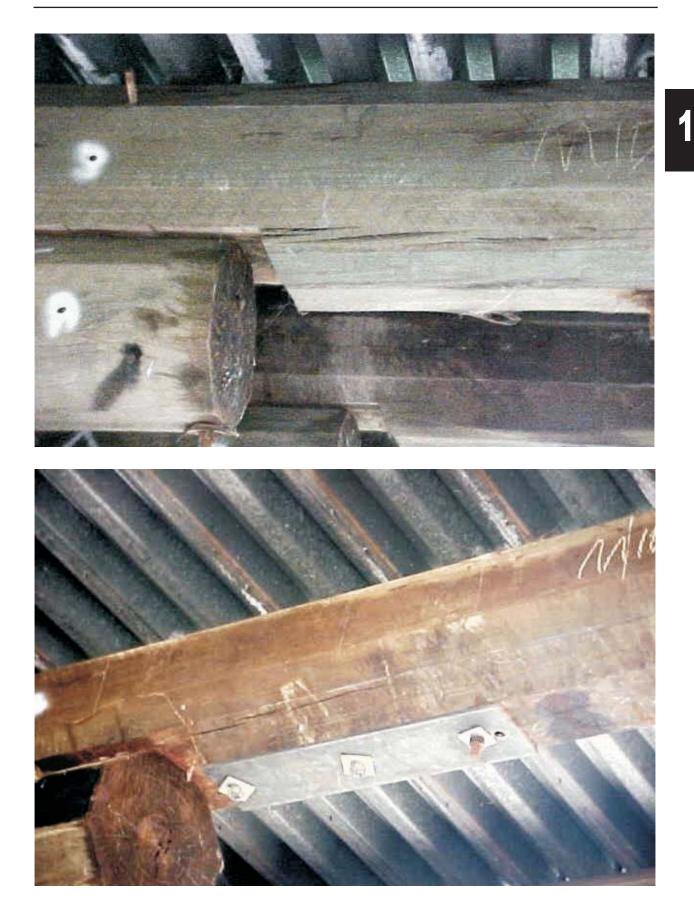
Figure 4.6(c) - Notch Cracking
