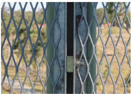
Note the use of expanded mesh – orientation may cause a louvre effect.
