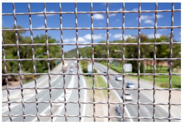
Figure 5.14(a) – Woven wire mesh with preferred 25 mm x 25 mm aperture
