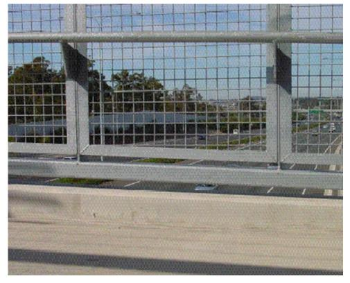
Figure 5.14(c) – Older screen with 50 mm x 50 mm x 4mm welded wire mesh
