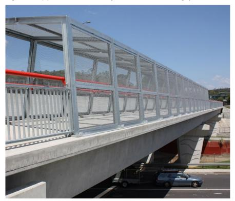
Figure 5.14(d) – Use of cover strips to close slots and gaps
