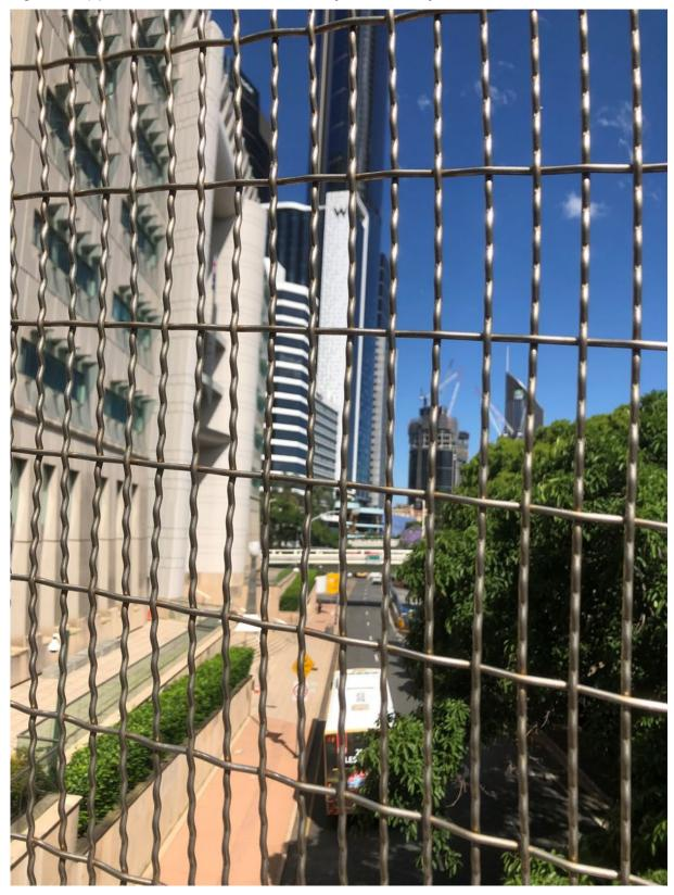
Figure 5.14(b) – Woven wire mesh with vertically orientated aperture
