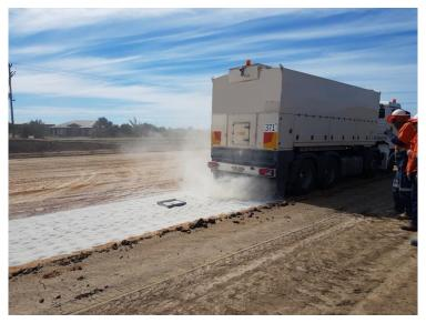
Figure 4.9.7.6(b) – Slaking of quicklime
