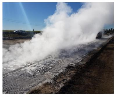
Figure 4.9.7.6(d) – Steam cloud generated during slaking of lime
