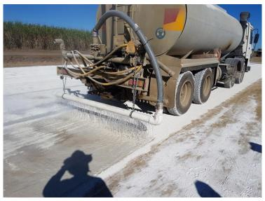
Figure 4.9.7.6(c) – Slaking of quicklime
