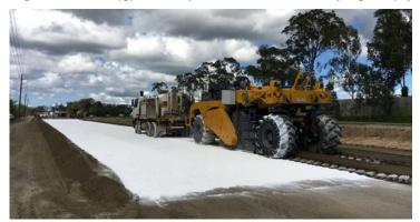
Figure 4.9.8.6.1(h) – Light compaction (smooth drum) of bulked material
