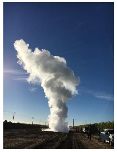
Figure 4.9.7.6(e) – Lime stabilisation of an expansive-soil subgrade in the outer region of a pavement
