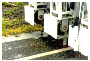
Figure 4.9.7.7(e) – Injected lime under pressure exiting through cracks in the pavement
