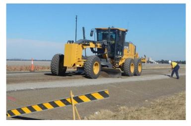
Figure 4.9.8.6.1(j) – Target depth needs to account for the bulked height above finish surface level
