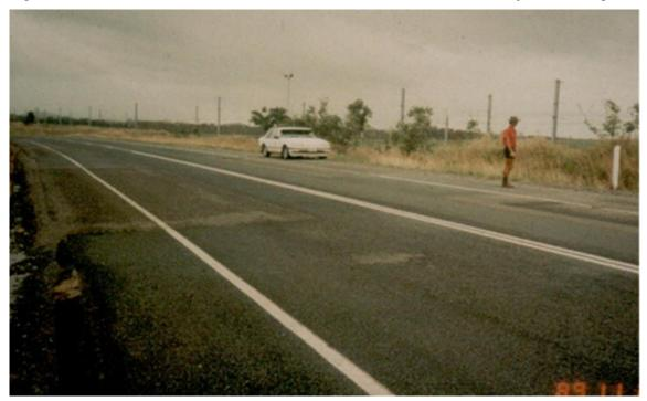
Figure 2.13.10.5 – Failures as a result of 'boxed' construction with inadequate drainage
