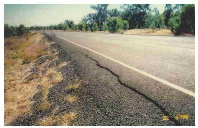
Figure 4.9.7.1.2(b) – Longitudinal cracking of a cementitiously treated base on an expansive soil embankment
