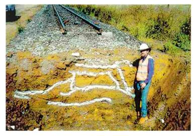
Figure 4.9.7.7(c) – The creation of a 'lime curtain' formed via injection of lime
