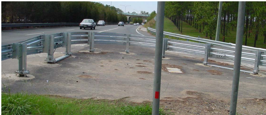
Figure 8.51 Thrie beam bullnose installation
