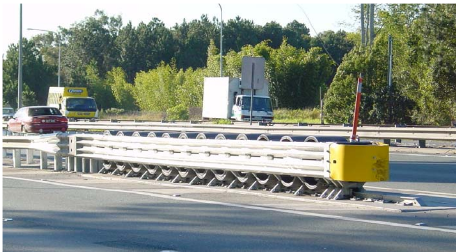
Figure 8.55 End treatment - "QuadGuard Elite" system
