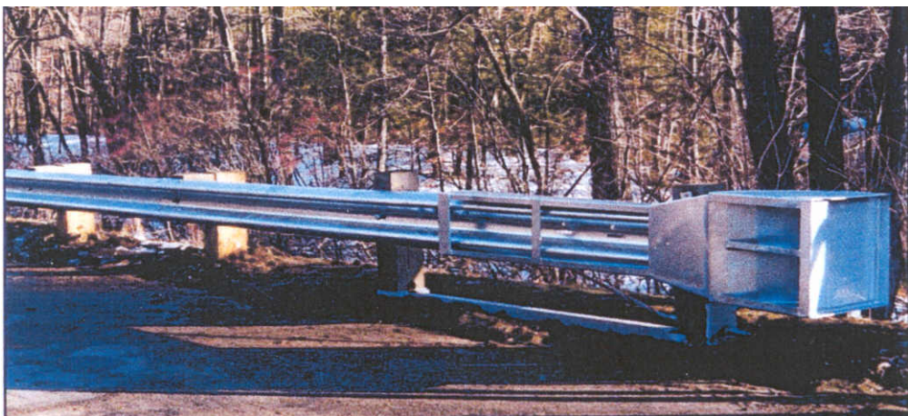
Figure 8.46 Example of SKT installation
