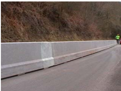
Figure 8.64 BarrierGuard 800 (Test Levels 3 and 4)
