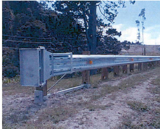
Figure 8.47 Example of FLEAT installation
