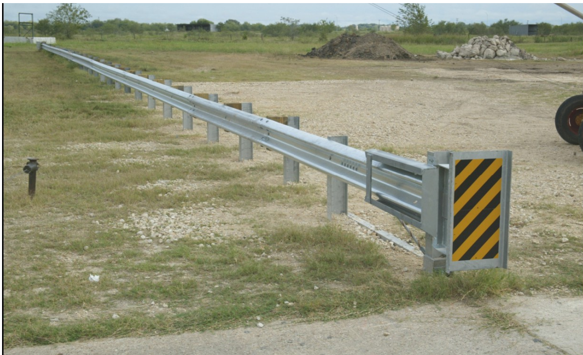
Figure 8.48 Example of ET2000 Plus installation
