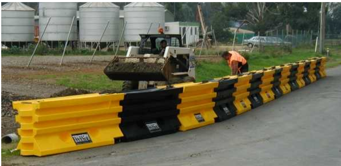
Figure 8.61 The Triton® barrier (Test Level 0)
