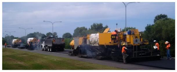
Currently, the department does not have a standard specification for HIPAR. Transport and Main Roads' *Pavement Rehabilitation Manual* (Section 4.4.14) provides guidance on the use of HIPAR including the required materials and design considerations.
