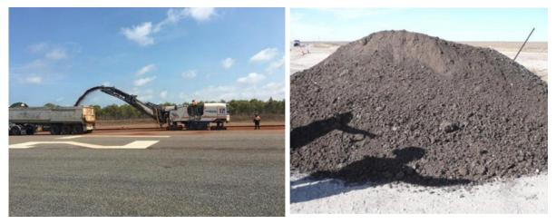
Current Transport and Main Roads specifications allow the incorporation of RAP into dense graded asphalt mixes for surfacing, intermediate, base and corrector courses. <u>MRT30 Asphalt Pavements</u>, <u>MRTS32 High Modulus Asphalt (EME2) and MRTS102 Reclaimed Asphalt Pavement Material</u> set out the requirements for RAP that is used in asphalt.
