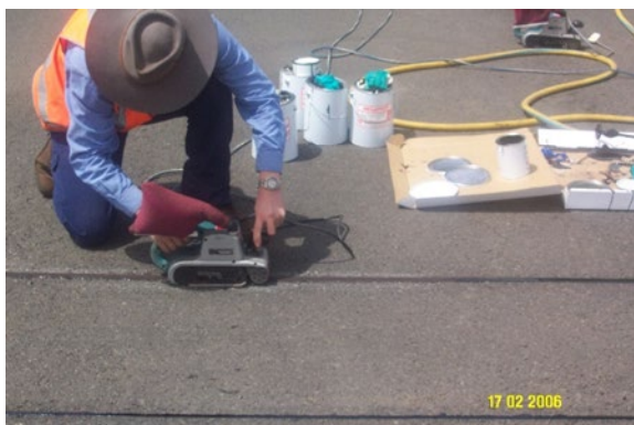
Figure 7.4.4(h) – Piezoelectric installation details (making epoxy level with road surface)
