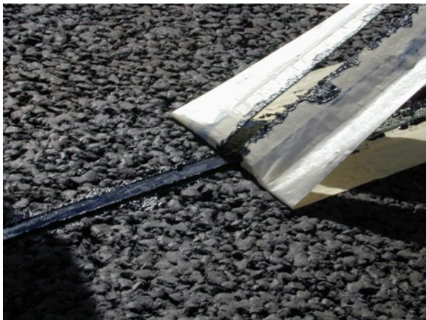
Figure 7.4.4(g) – Piezoelectric installation details (removal of sealant excess)
