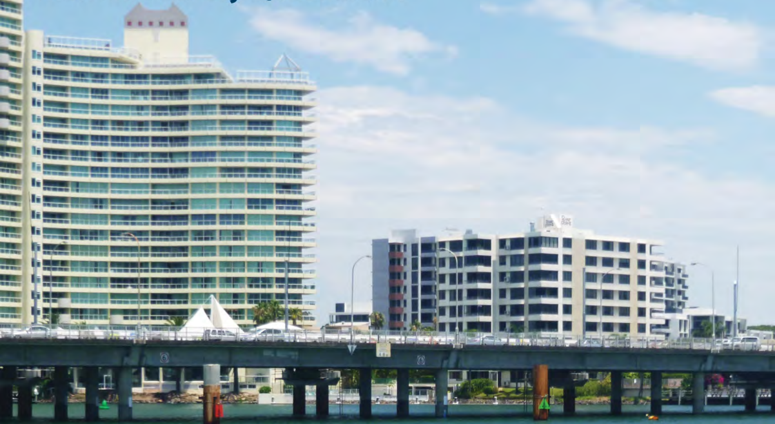
Gold Coast Bridge, Nerang River
