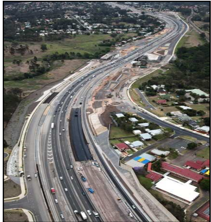
Eastbound motorway construction in Redbank
