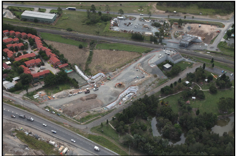
Bridge works at Monash Road, Redbank.
