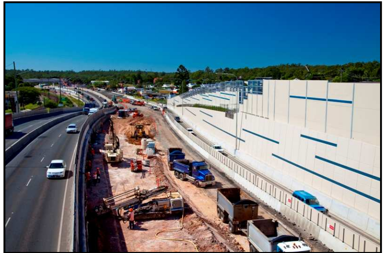
Construction of the new motorway alignment at Goodna
