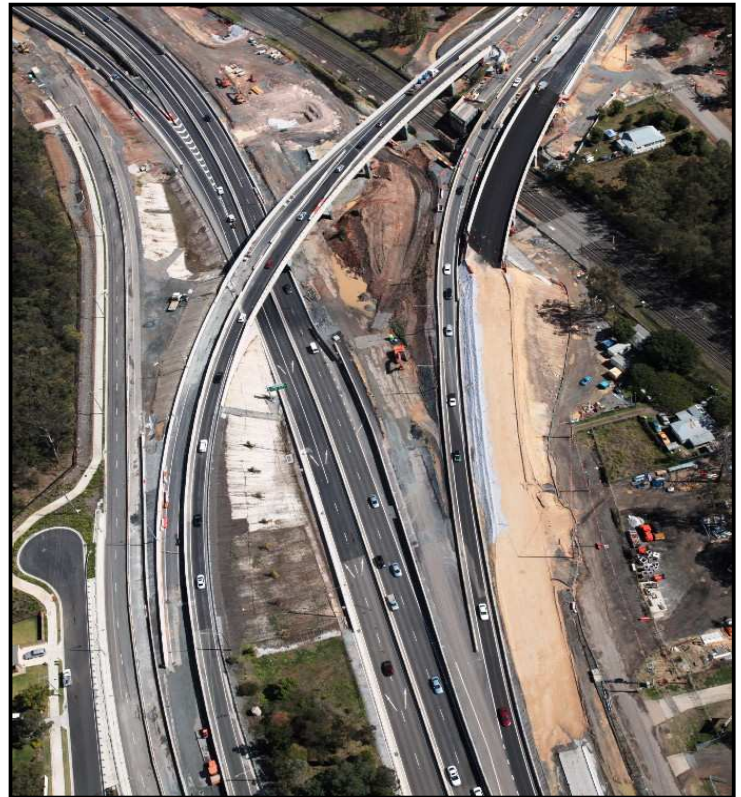
The Warrego off-ramp and new bridge construction in Dinmore
