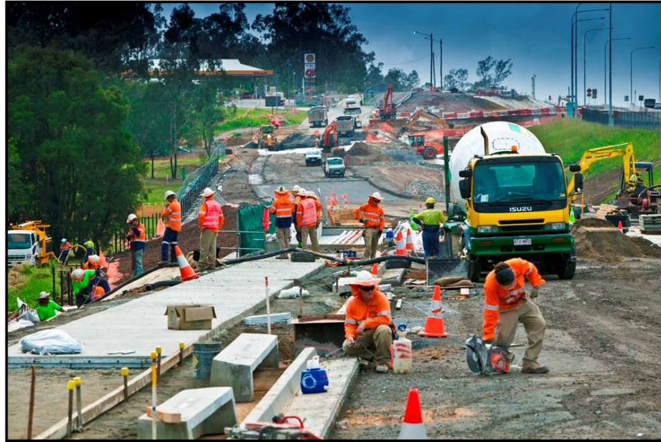
Works on the new service road at Redbank
