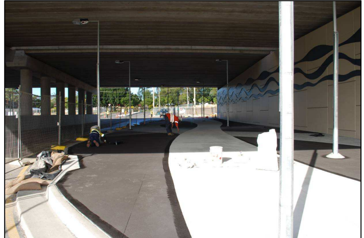
Painting underway on the Endeavour Road connection footpath
