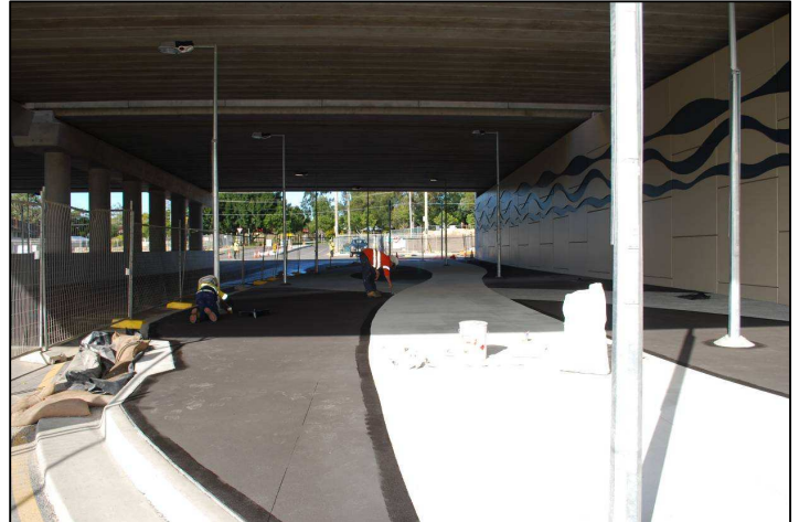
Painting underway on the Endeavour Road connection footpath
