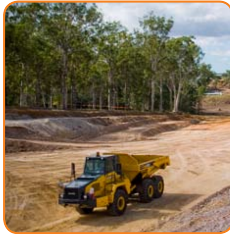
Earthworks along the Ipswich Motorway.
