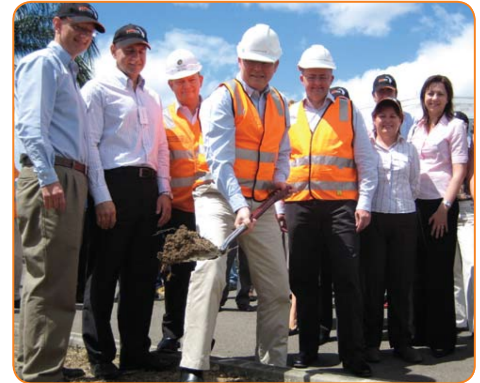
Prime Minister Kevin Rudd turns the first sod of the upgrade, beside federal, state and local representatives.
