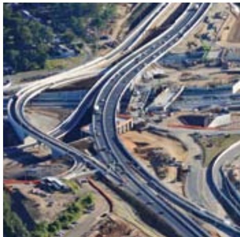
The Centenary Highway Interchange now free-flowing and almost complete
