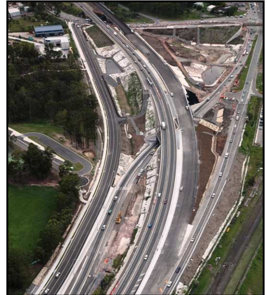
Westbound view of works at the Dinmore end of the project
