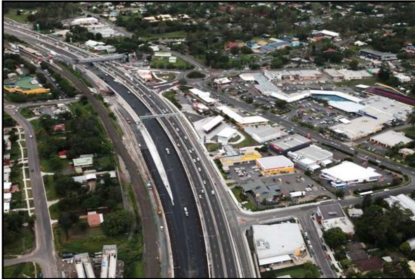
Eastbound view of works at the Goodna end of the project
