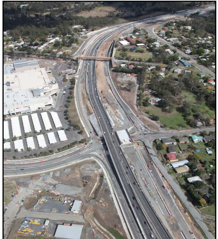
Construction of the new Brisbane bound motorway lanes through Redbank
