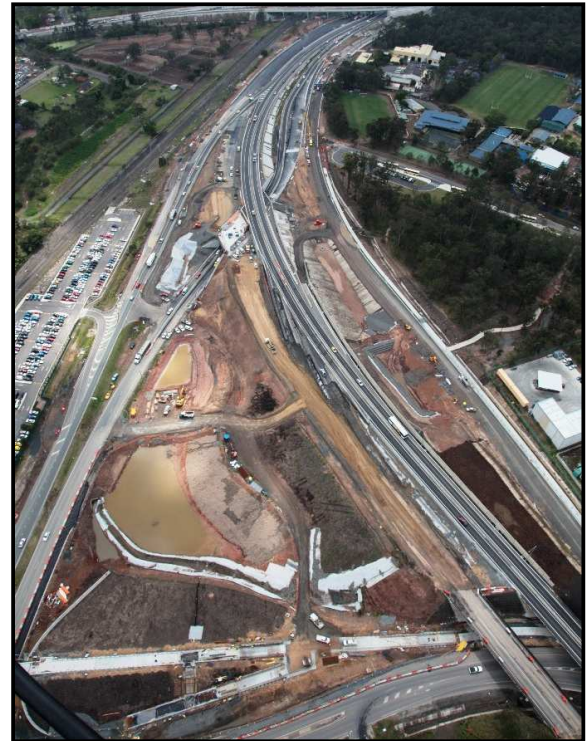
Works in Dinmore including construction of the new Dinmore pedestrian bridge
