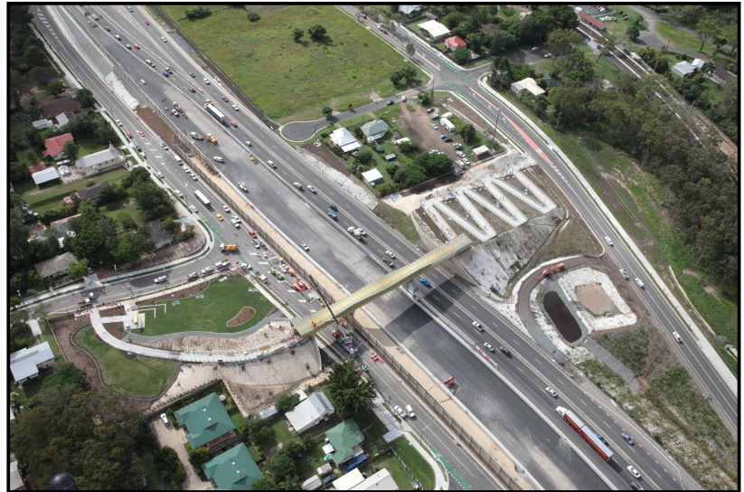
The Tessman Street pedestrian bridge in Riverview is now complete
