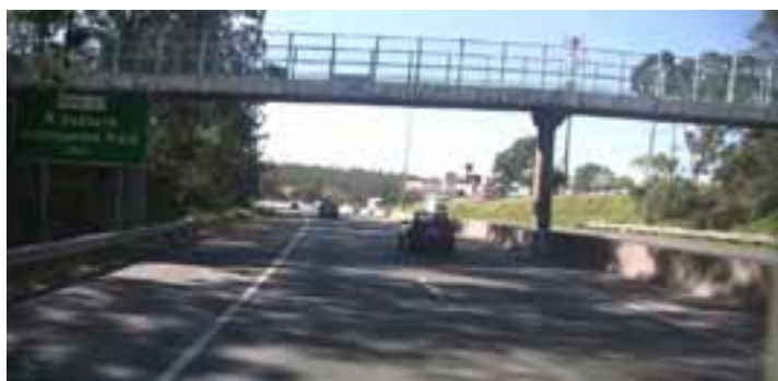
Old pedestrian bridge at Law Street – 2008
