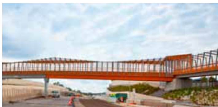
New pedestrian bridge at Law Street – 2011
