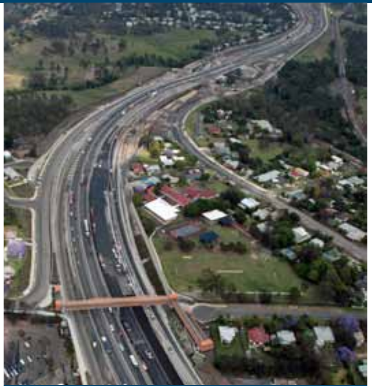
Looking west over Six Mile Creek – October 2011
