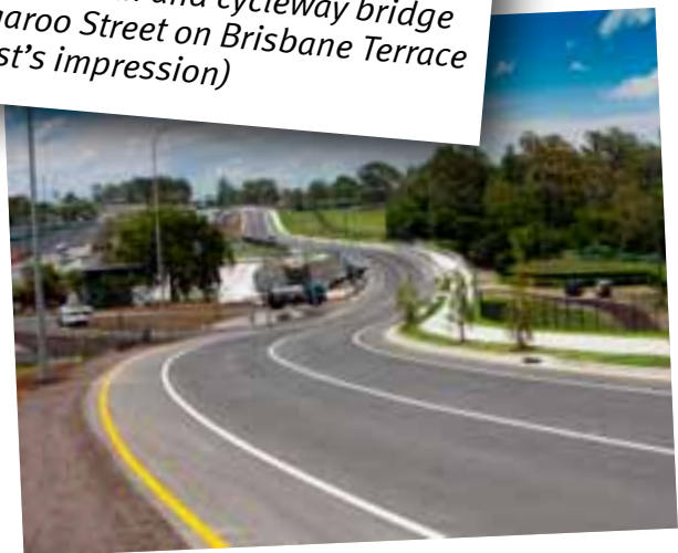
The new northern and southern service roads alongside the motorway were recently opened to traffic
