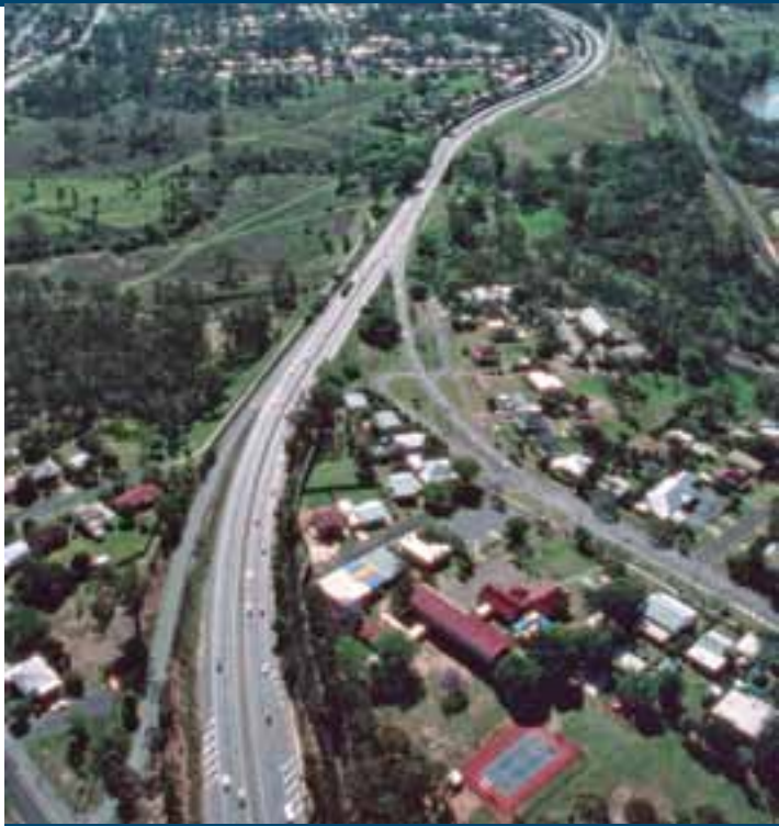
Looking west over Six Mile Creek – October 2008
