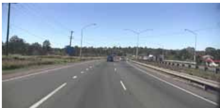
Old motorway at Six Mile Creek – 2008
