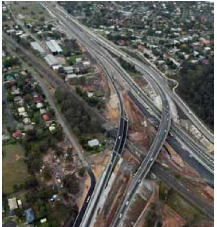
Looking east over Warrego Highway – October 2011
