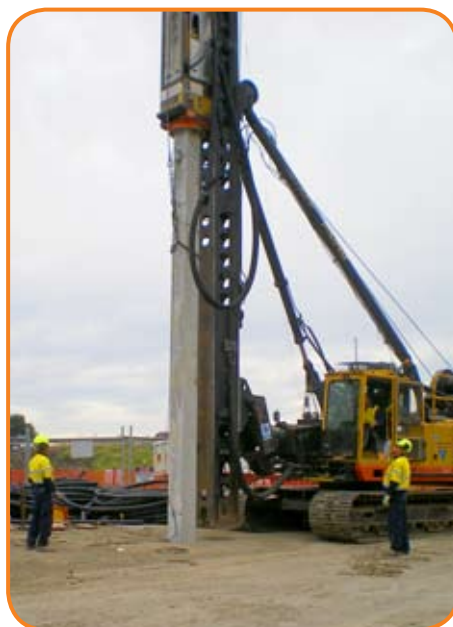
An example of driven piling, courtesy of Wagstaff Piling.
