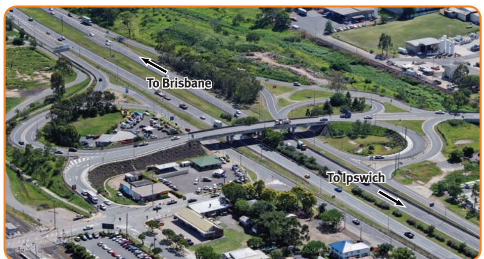
Service interchange: Progress Road Interchange at Wacol.
