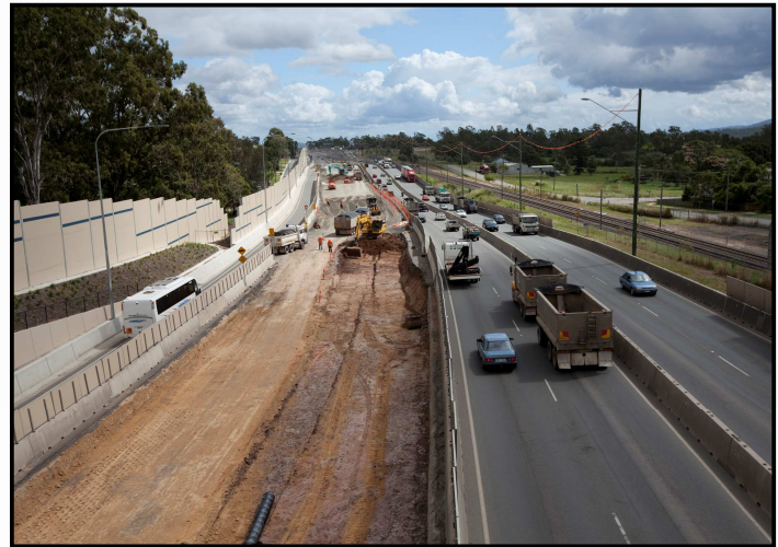
New motorway construction at Goodna (westbound)
