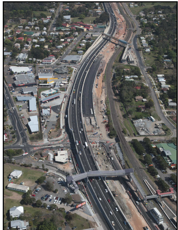
Construction in the Goodna area is progressing well
