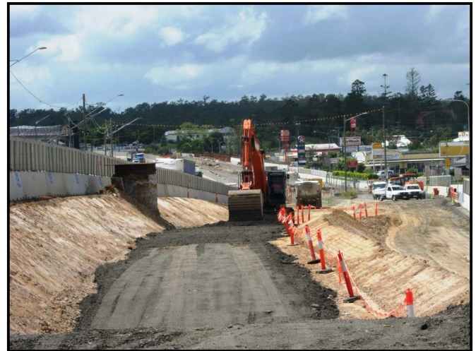
Construction works on the Ipswich Motorway at Goodna
