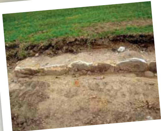
Old kerbing at Redbank
