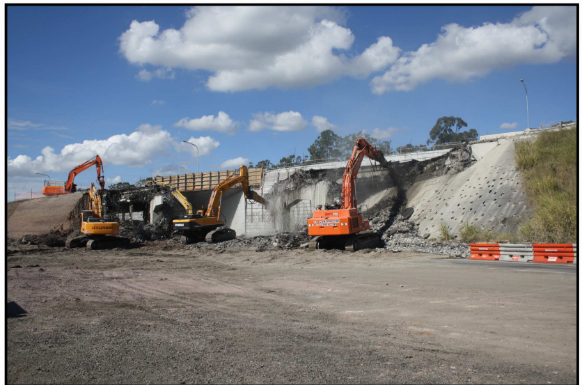
Old Cunningham Highway bridge demolition in Dinmore
