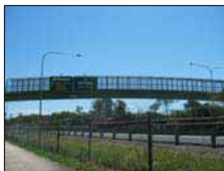
A pedestrian bridge with caging
