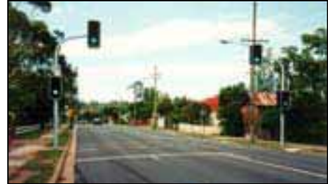
Pedestrian actuated traffic signals (mid-block)
