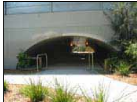
A high standard underpass
