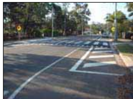
Chevron markings to deter parking
