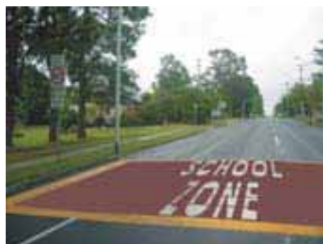
A typical threshold treatment
