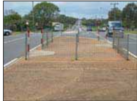
Pedestrian fencing on a median
