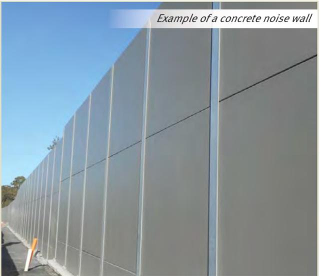
Example of a concrete noise wall
