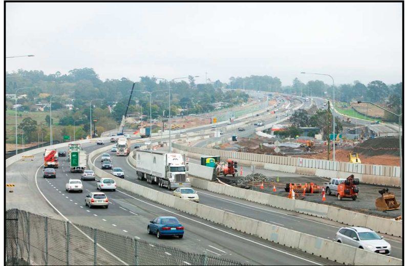
Works near Six Mile Creek
