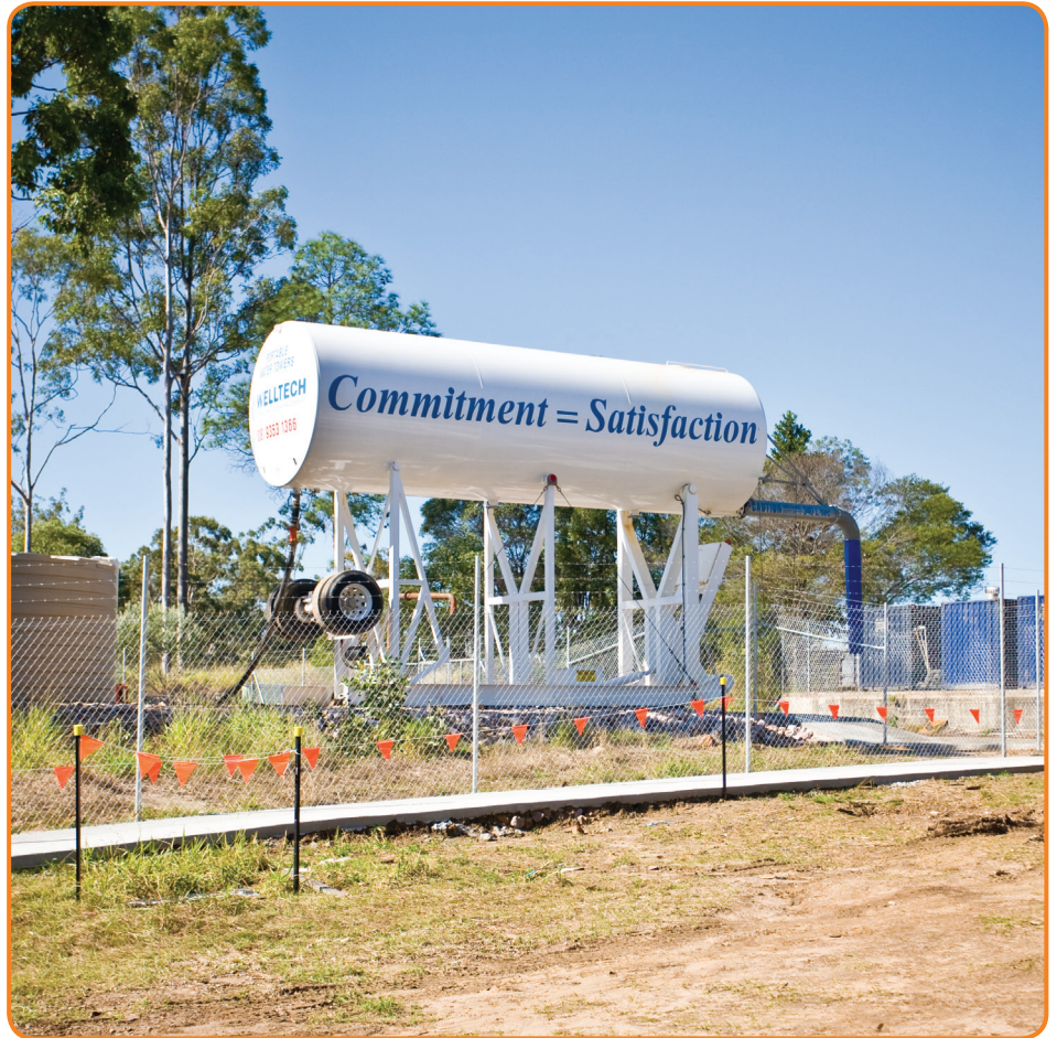
Recycled water is used throughout construction.
