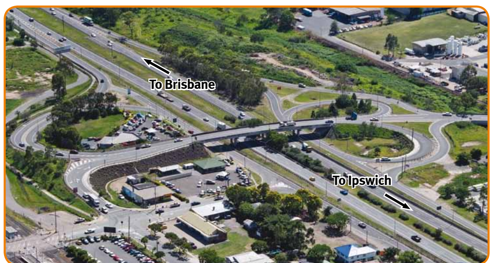
Service interchange: Progress Road Interchange at Wacol.
