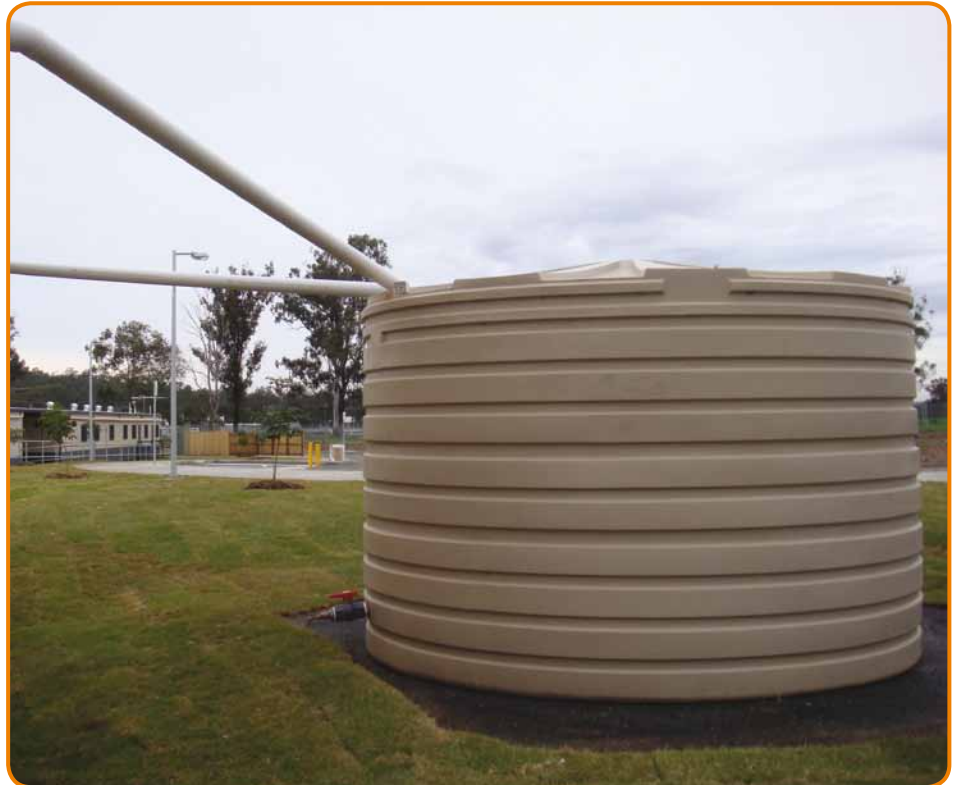
Water tanks are used during construction to capture rain water to reuse on site.
