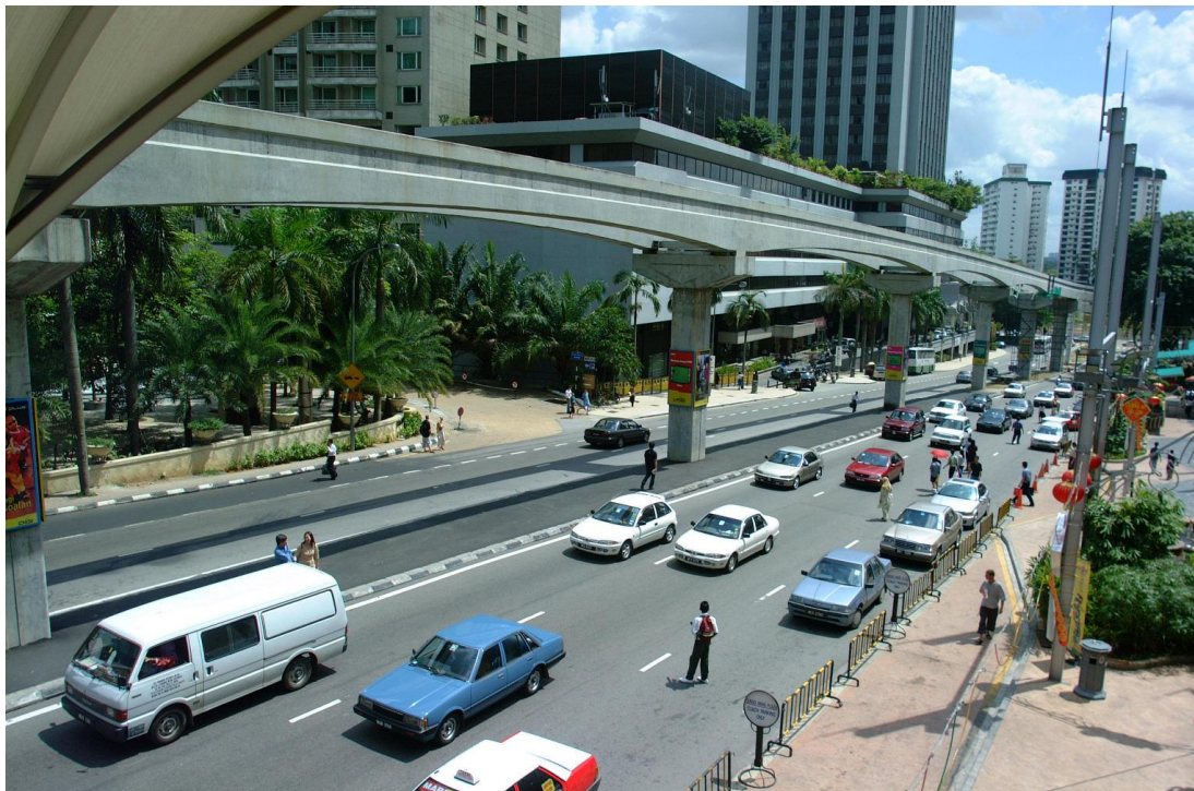
Figure 7-5: Centre median rail line, Kuala Lumpur (source: Wikimedia Commons)
