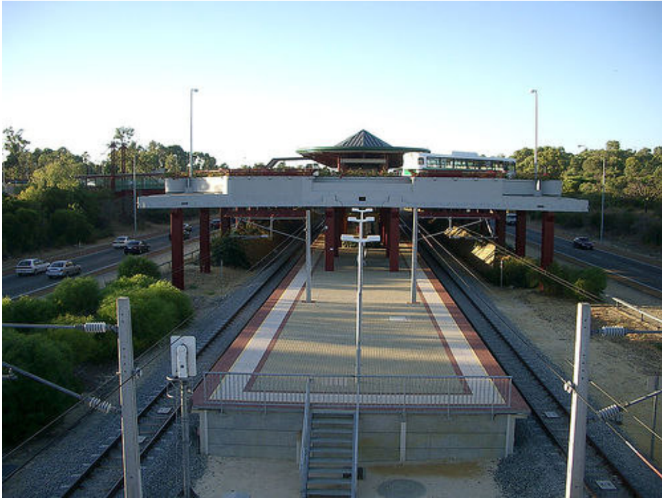
Figure 5-11: Bus/rail interchange at Whitfords, Perth
