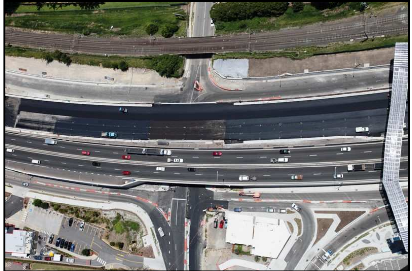
Left – Looking westbound over the Ipswich Motorway at Goodna Above – the Church Street underpass at Goodna
