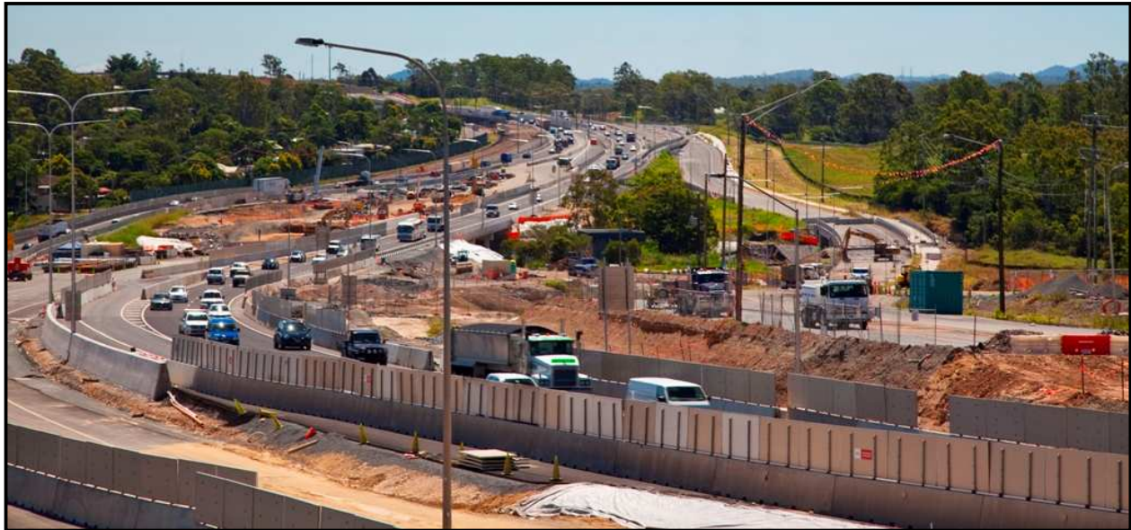
Construction works at Six Mile Creek, Riverview
