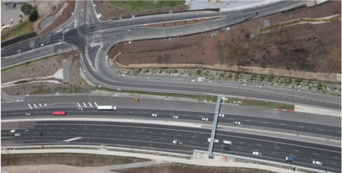
An aerial shot of Redbank showing the Ipswich Motorway and the new Francis Street and Brisbane Road intersection.
