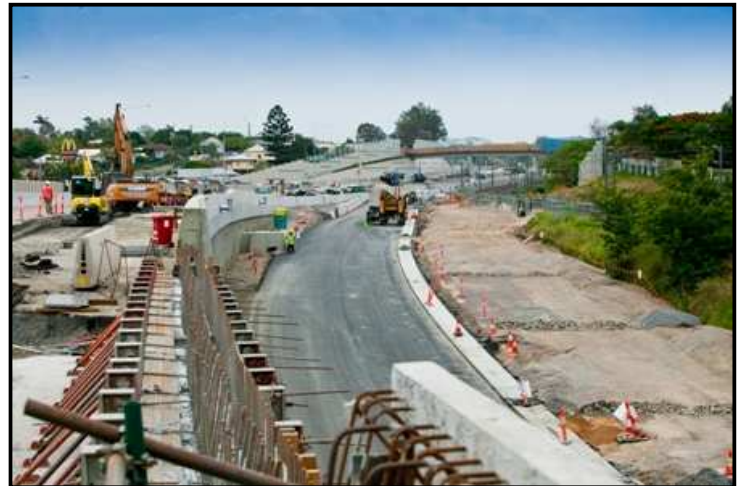
The new Church Street off-ramp in Goodna is under construction
