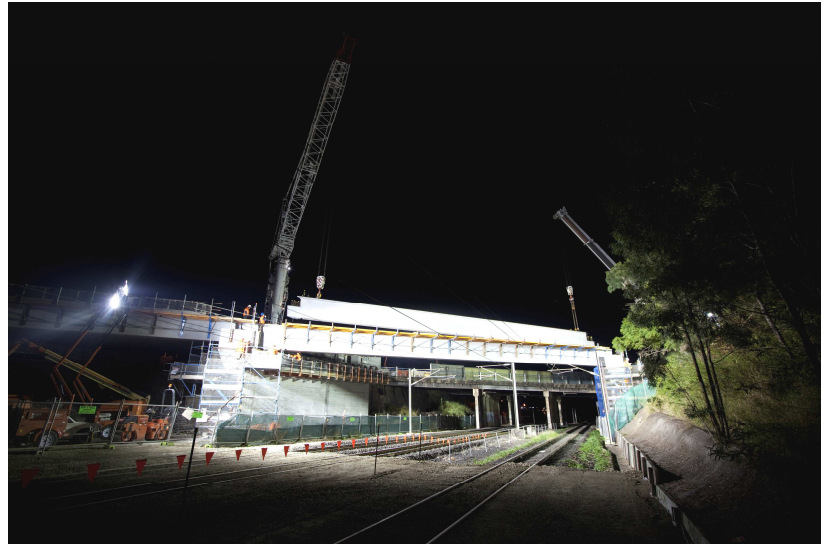
Bridge deck lift for the Warrego Highway eastbound bridge
