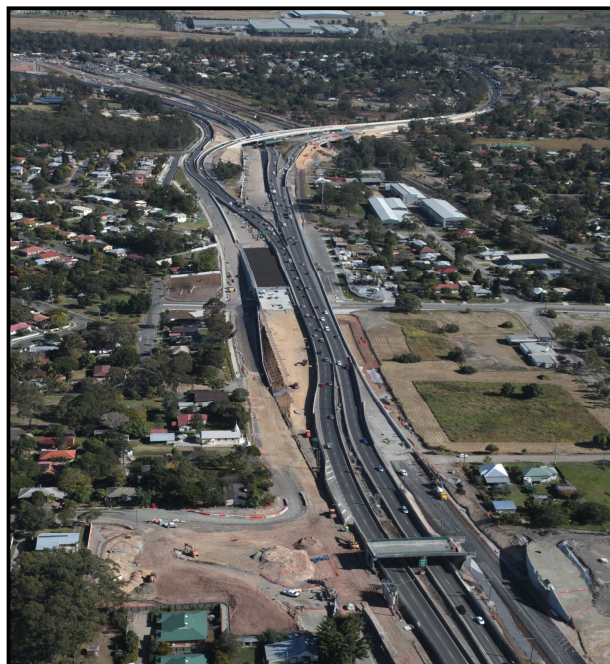
Works at the western end of the project
