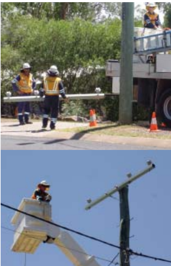
Figure 1 : Cross-Arm Installation
