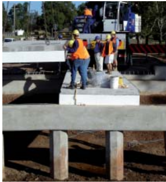
Figure 7 : Wagners CFT Bridge Installation
