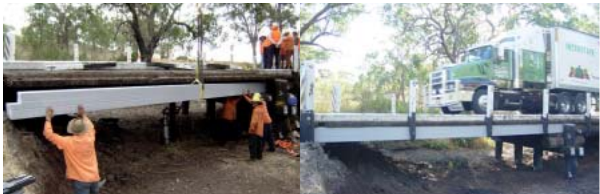
Figure 4 : Beam installation & working under load
