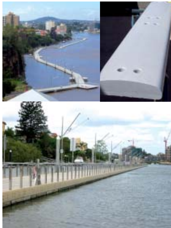
Figure 2 : FCDD's fibre composite Waler in the Brisbane City Wharf Project
