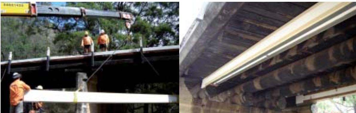
Figure 6 : Installation of FCDD Girder
